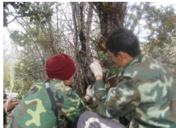
Fig.4 Install infrared surveillance camera
