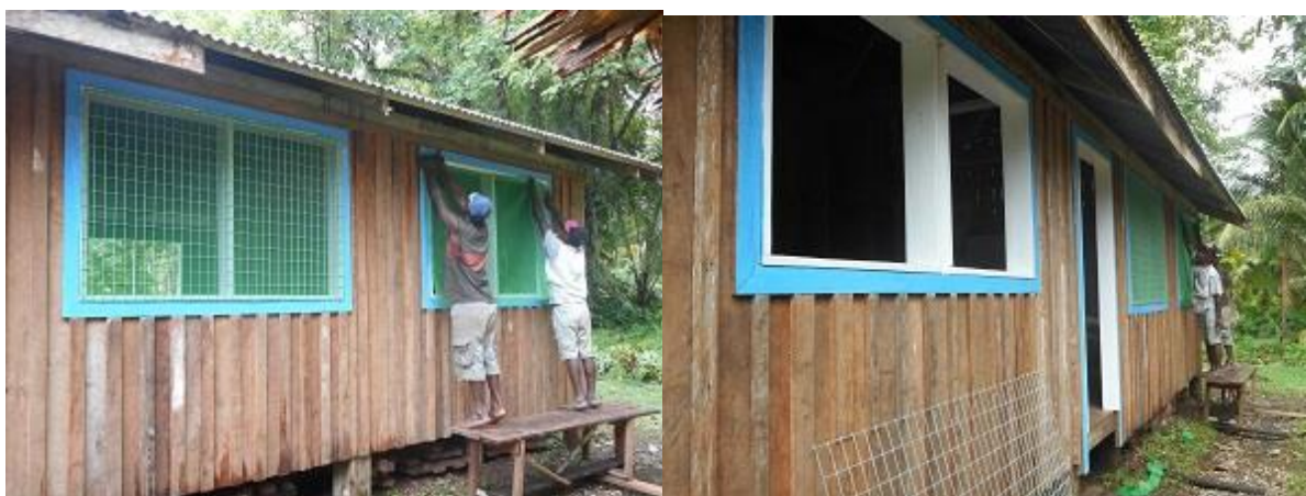
Installing windows to the conservation centre 300px
