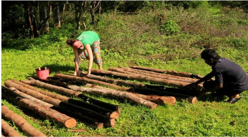
**Figure 4.7.** Painting fence posts with old engine oil to protect from termites – researcher Kylie M. Butler and field assistant Supun Herath © Morgan Tipper.
