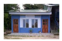
The fifth stage was the ceiling, divisions, tiled floor and painting which cost Q4000 for plywood, lamps, and wood for the ceiling, Q2000 for the paint, and Q7,000 for the tiled floor.
