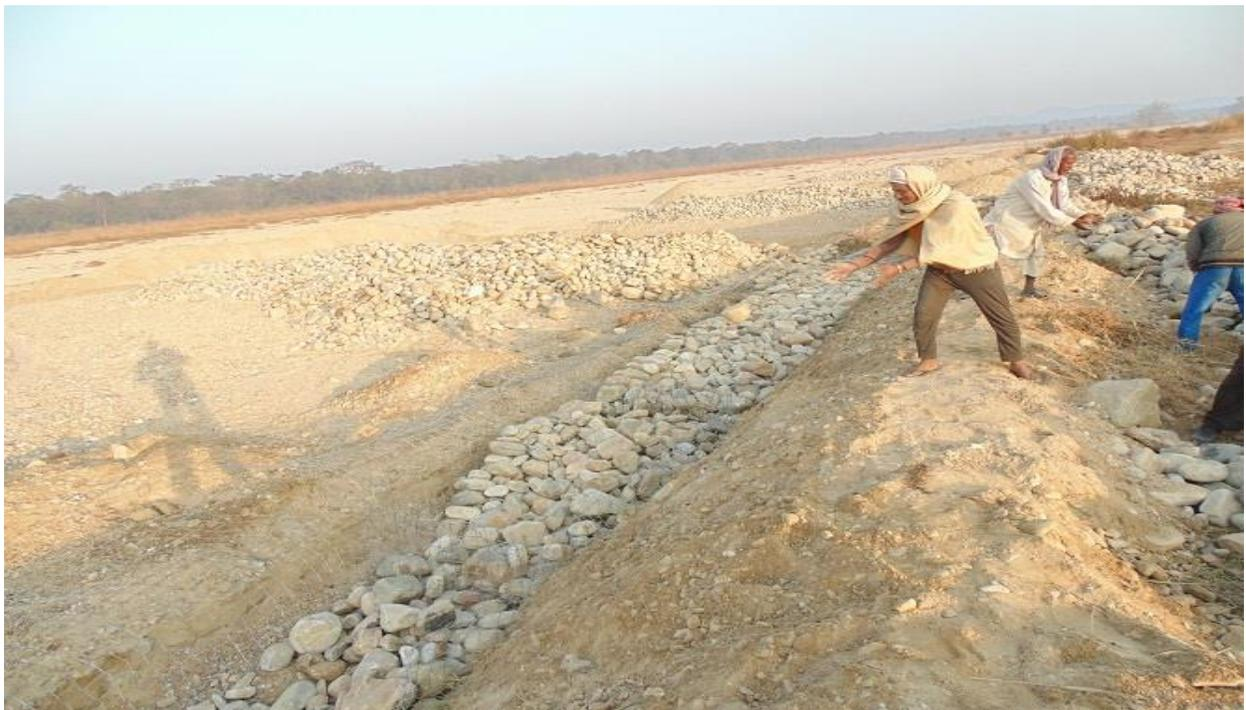
Fig. 12. Construction of Gabion box defences on the Bhata River to protect the banks from erosion.
