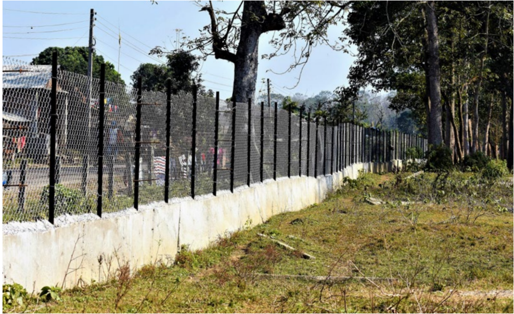
Figure 5.7 An example of the mesh wire fence communities prefer to construct along the forest-settlement border. The fence has a concrete base of about 2 feet and 5 feet tall mesh wire anchored to the iron poles set in a concrete base.
