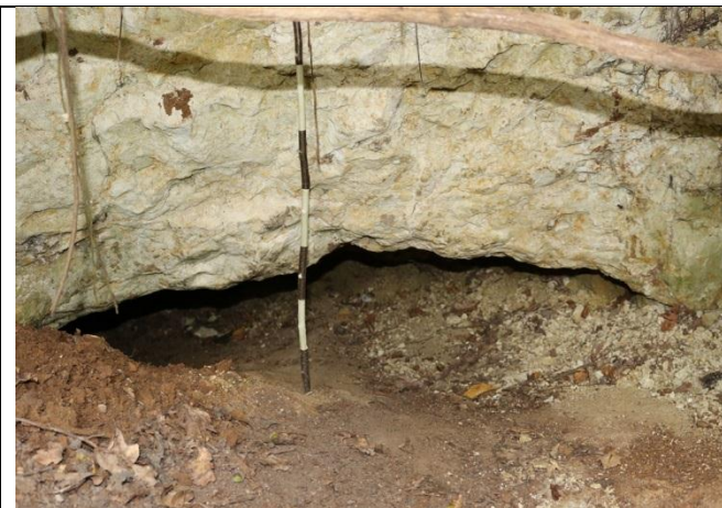
Liptsy 1 mine, entrance 2, close view (one section of the stick is 10 cm) in August 2017 (picture by Hukov V.)
