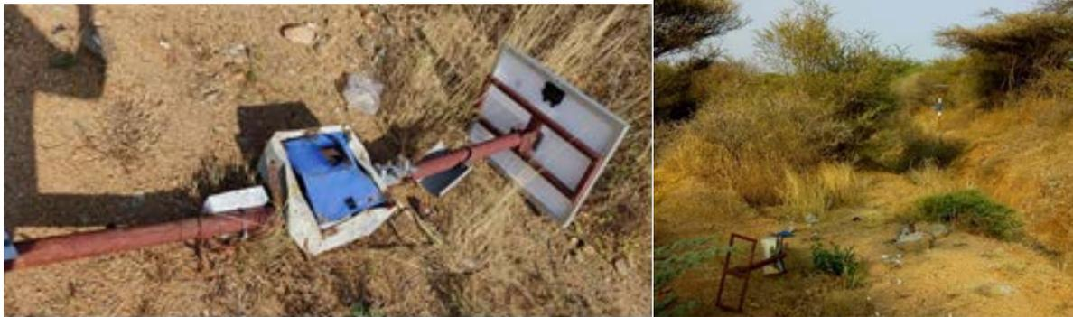
Fig. 3: Pole totally damaged by elephant. Fig. 4: Restored pole at farther distance after trench which is presently inaccessible by the elephants.
