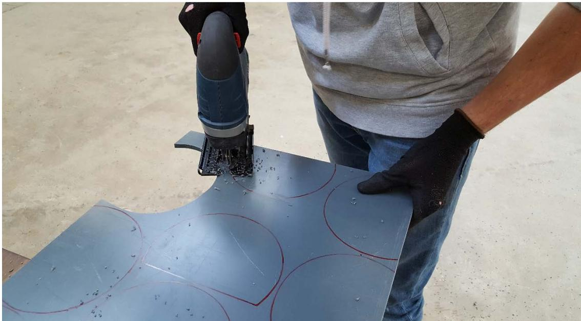
By making use of a jigsaw, very specific shapes were cut from thick (8mm) PVC sheets. These shapes are used within the larger 160mm diameter silos as a rooftop for individual plants. It ensures that collapsing soil does not injure the plants during growing and contamination stage.
