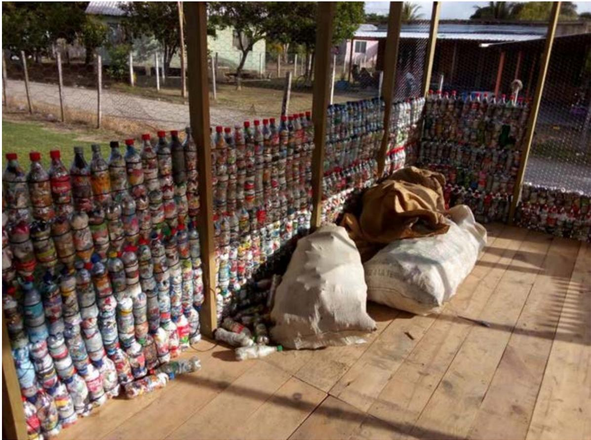
Once all the walls are filled with ecobricks, they will be covered with a layer of cement that will protect the chicken wire against the salt of the ocean
