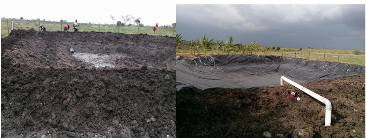
Left: Compaction of the soil to ensure stability. Right: Installation of water inlet into the pond.
