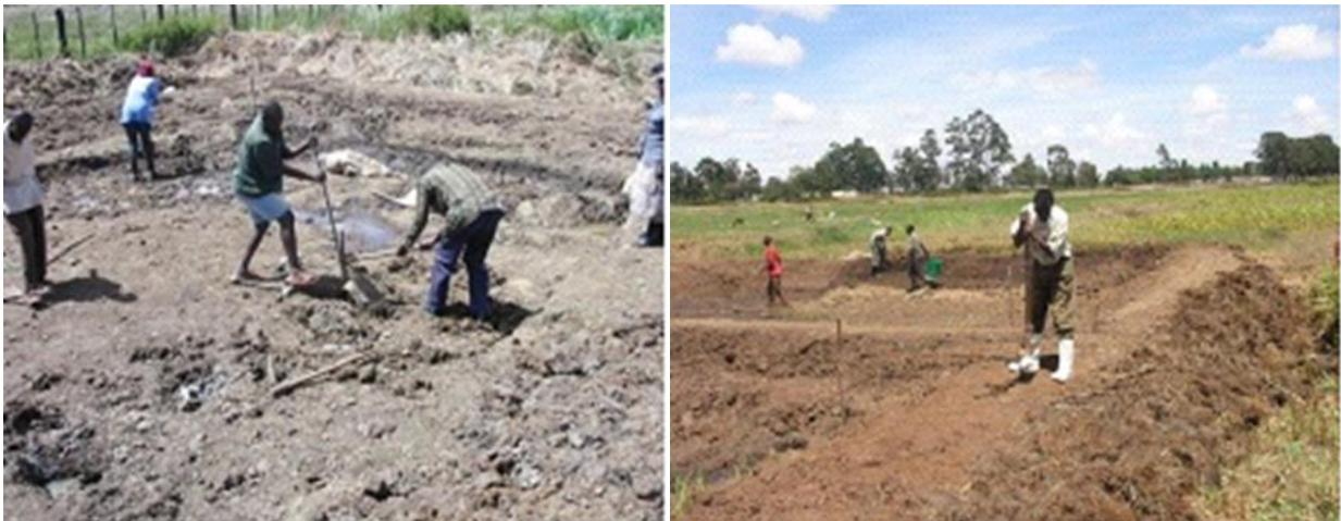
Left: Removal of boulders and the stumps from pond area. Right: Digging of trench all round within the dyke position to help prevent porosity
