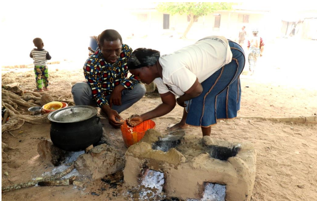
Training on how to maintain the cookstove by plastering cracks wall with clay
