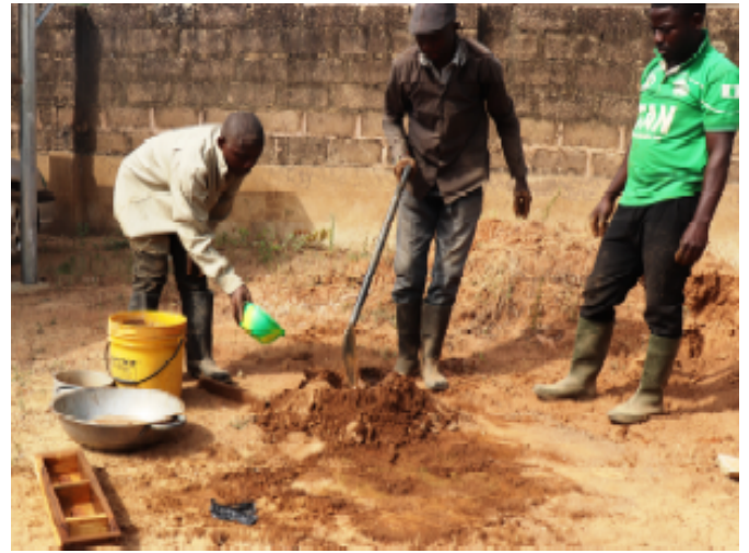
Left: Wooden mould use for production of clay blocks (©Fola Babalola). Right: Mixing of clay, topsoil, manure and sharp sand with water by members of project team (© Fola Babalola).
