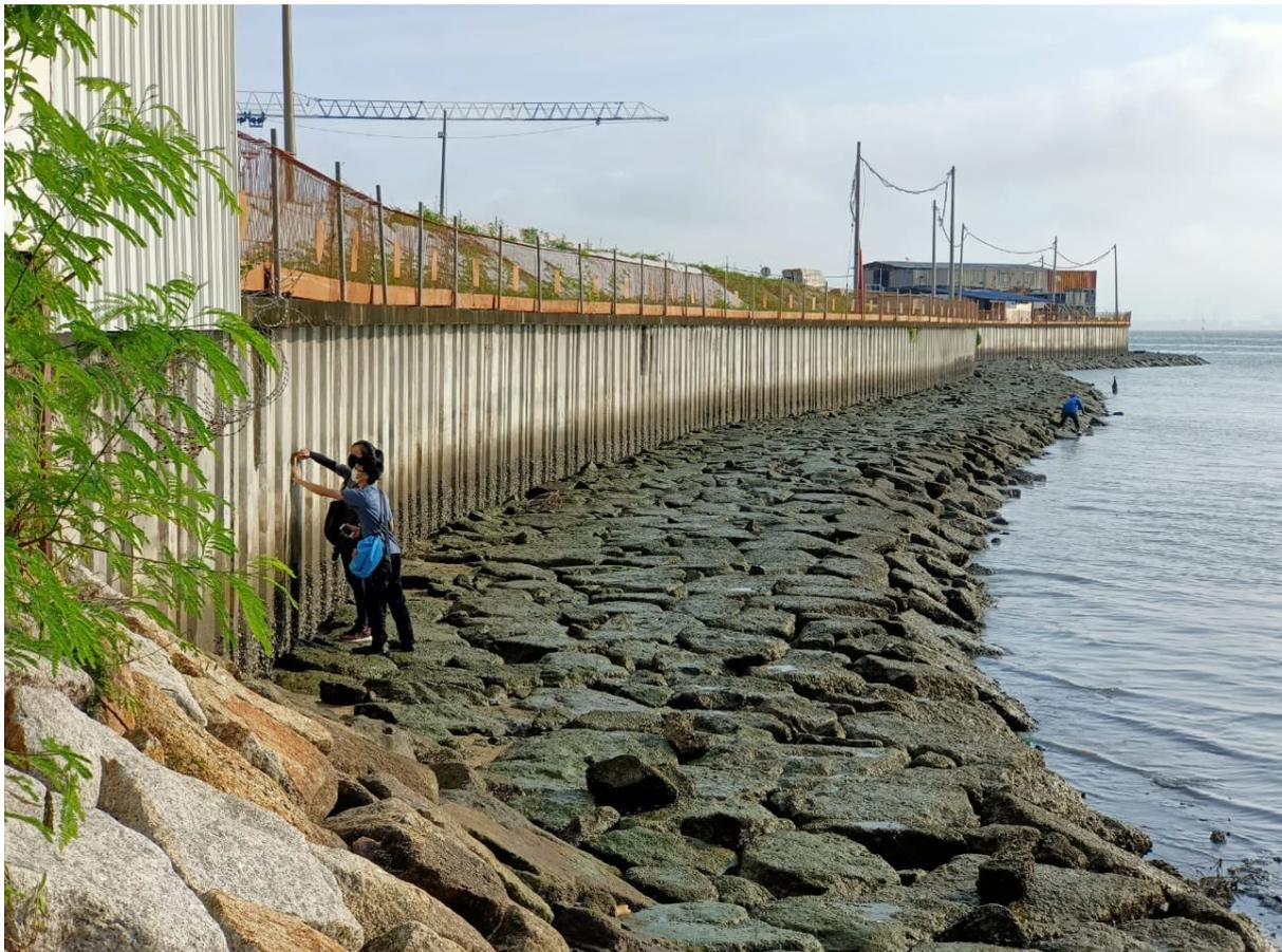
Fig. 7. Seawall at the new project location. Experimental tiles will be installed in the recesses of this wall and monitored for 9 months for its ecological enhancement capabilities.
