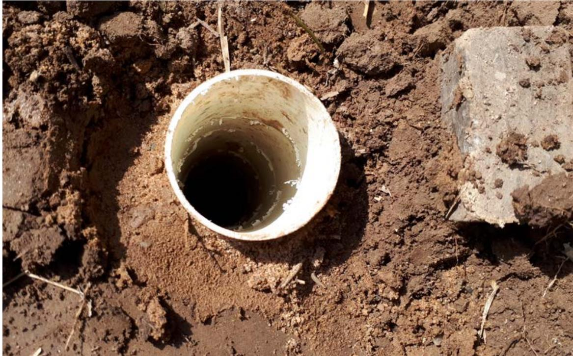
Photo 1. The hole made for the freatimeter is 3 m deep and 0.08 m diameter. The tube of the freatimeter has a 0.05 m diameter. Between the walls of the hole and the tube of the freatimeter is filled with sand that fulfils the function of filter.
