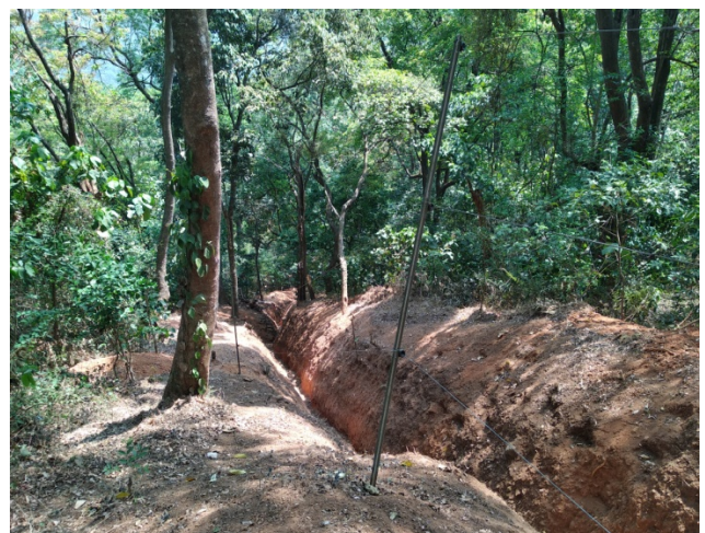
Fig 4. Elephant Proof Trench and fence erected on the boundary of village and forest.
