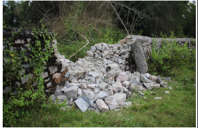
Fig 2. A stone wall erected in the forest and village boundary is damaged by elephants.
