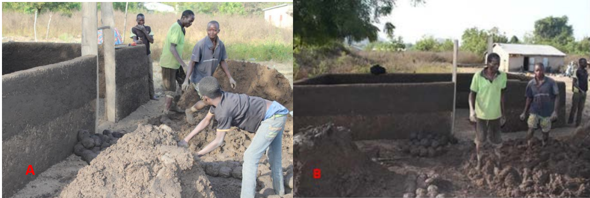
Photo 1: (A) and (B) Construction of the edible mushroom field based on rammed earth with the local populations in Wari-Maró.
