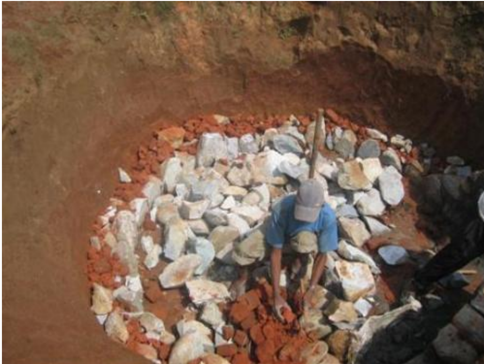
Construction of biogas plant in Bharkhore
