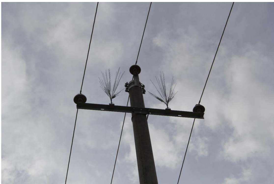
Figure 8. Perch deflector at the poles of 15kV line between Bayankhongor and Bayan-Ovoo villages. But all carcasses were found under poles with such deflector.
