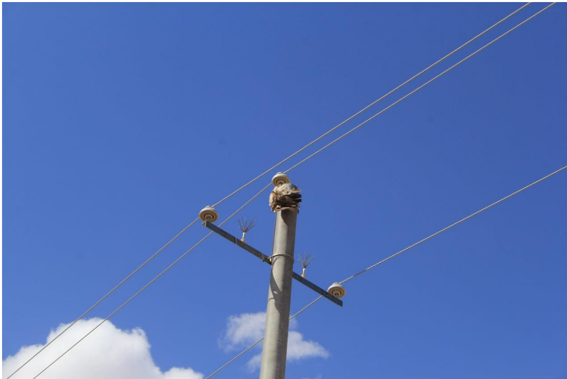
Figure 13. Saker falcon's carcass at top of the pole. Also this photo illustrated the types of perch deflector, which was relatively smaller.
