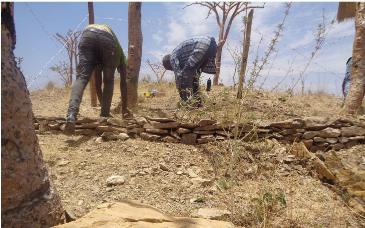
Figure 3. Introduction of soil and water conservation structures inside of the degraded of *B. papyrifera*
