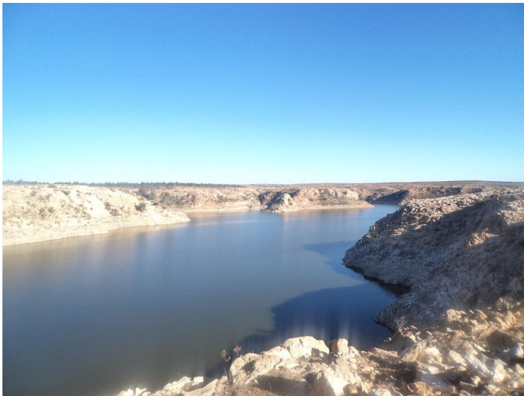
Figure 1: Topography of Mai-nefhi Dam
