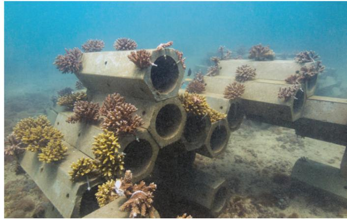
Photo 15: A MOSES-reef artificial structure patch at Mkwiro Community Managed Area. Its design provides a substrate for coral recruits and shelter and a hiding area for Octopuses, eels, and other camouflaging fish. Credit: Ewout Knoester
