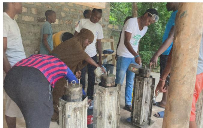
Photo 21: Participants engage in hands-on construction and filling in mixture in the MOSES-reef mold for MOSES-reef artificial structure. Credit: Cindy Saru
