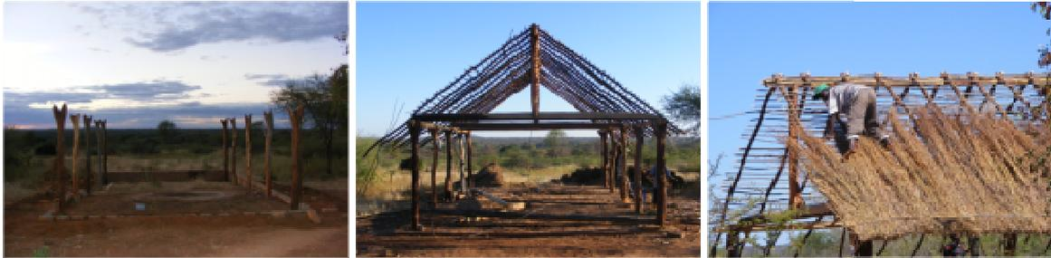
*Constructing and thatching the main shade banda at the new RCP field camp*
