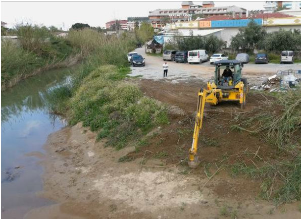
Fotoğraf 7. During restoration
