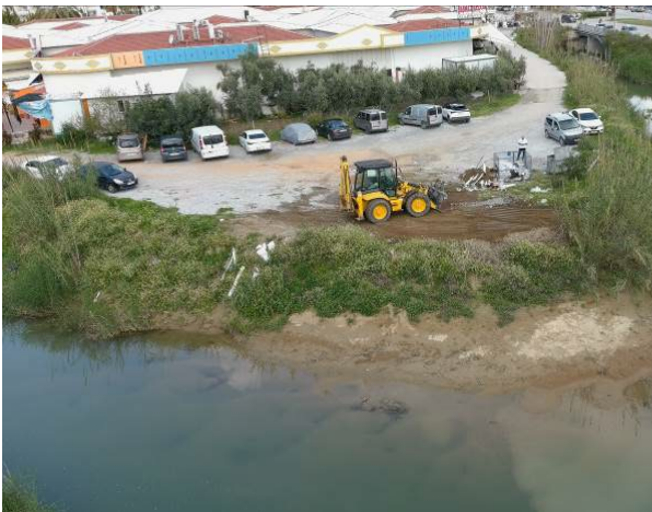
Fotoğraf 5. During restoration
