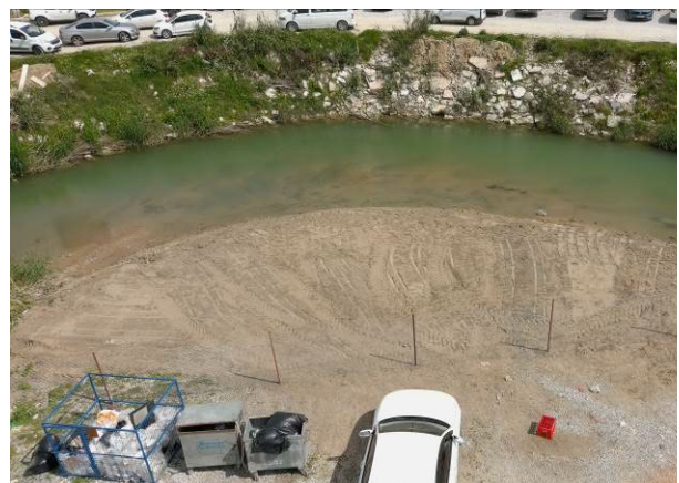
Fotoğraf 12. Installation of Protective Fencing
