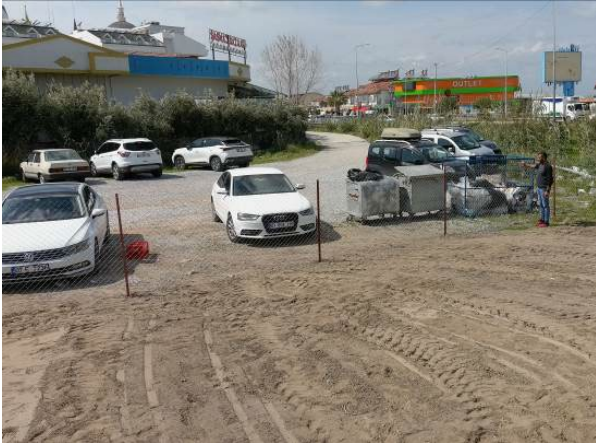
Fotoğraf 13. Installation of Protective Fencing
