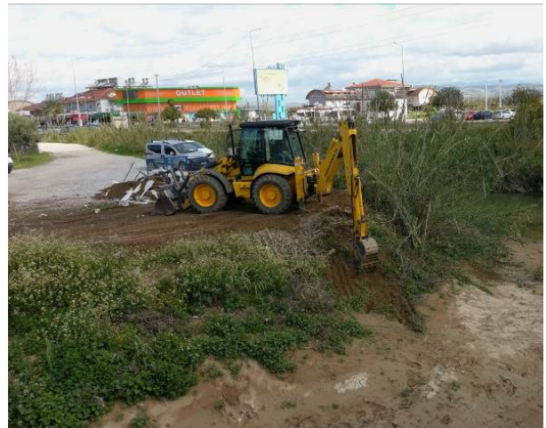
Fotoğraf 6. During restoration
