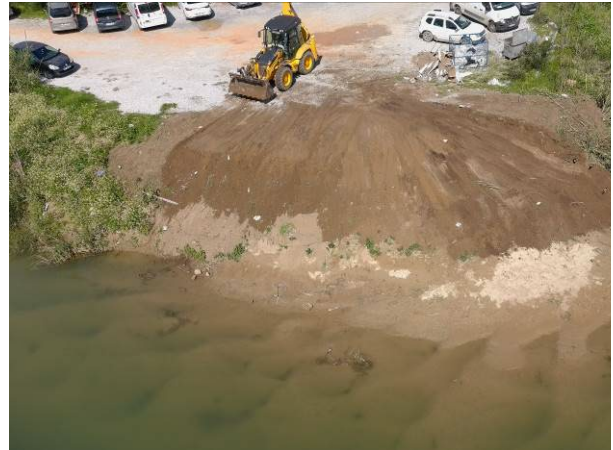
Fotoğraf 8. During restoration
