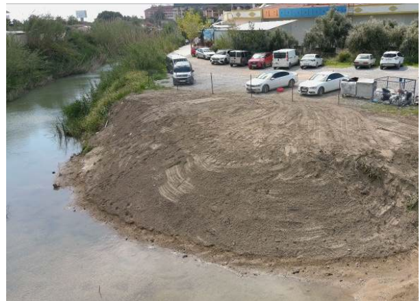
Fotoğraf 14. General View of the Restoration Area
