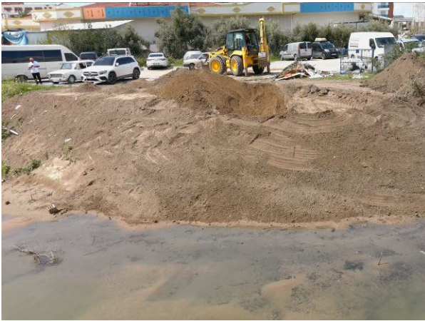
Fotoğraf 9. During restoration
