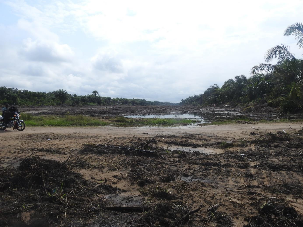
Fig. 1. Forest cleared to give way for the Lagos-Calabar coastal highway.
