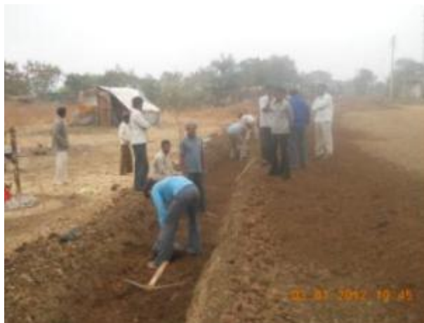
Figure 31: Eco-restoration work going on at Kajaleshwar village.
