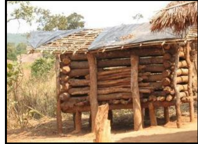
Effective design if it is well maintained has a strong door and log ceiling.
