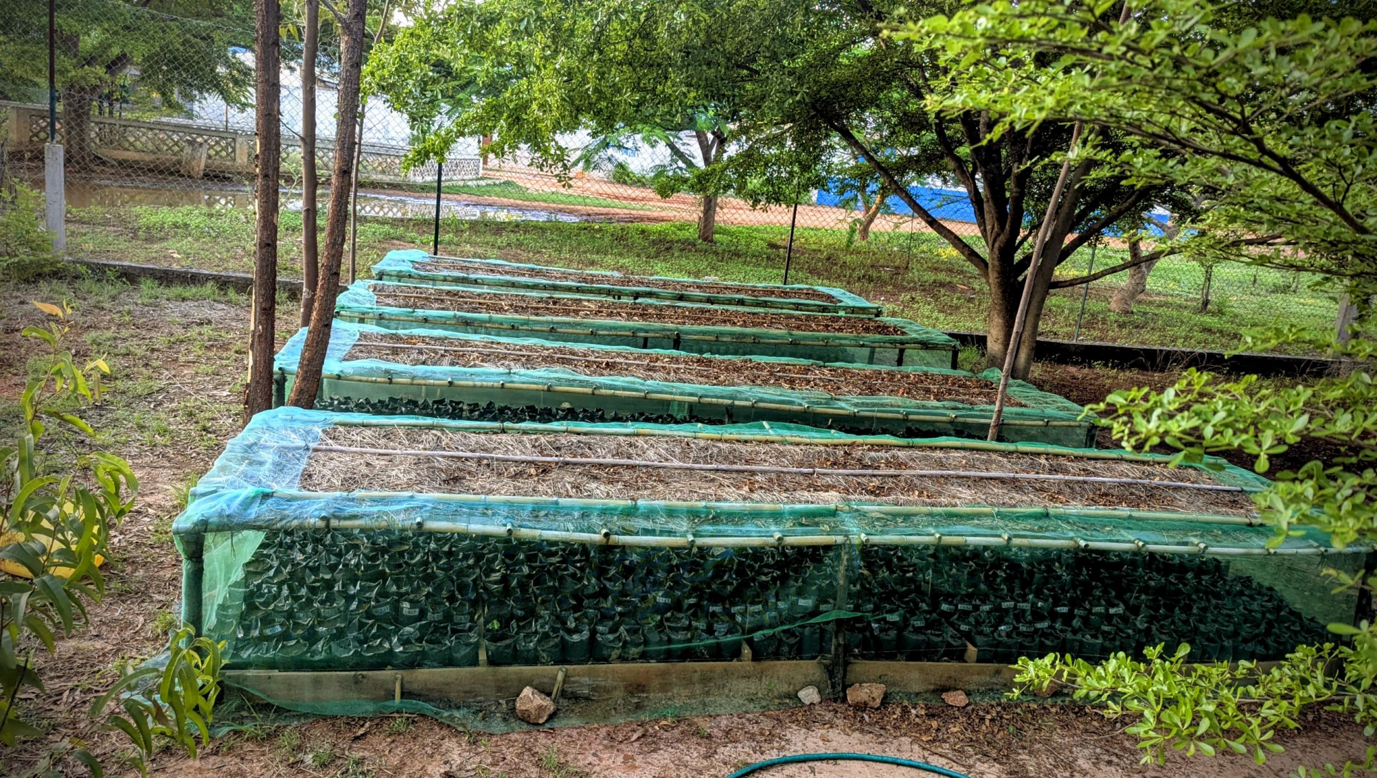
Installation of physical pest barriers
