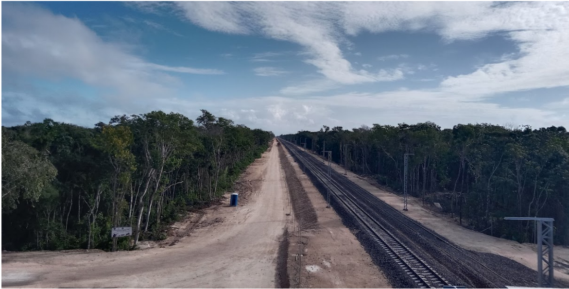
Figure 3. Progress on the construction of the Tren Maya railroad tracks during August 2024.
