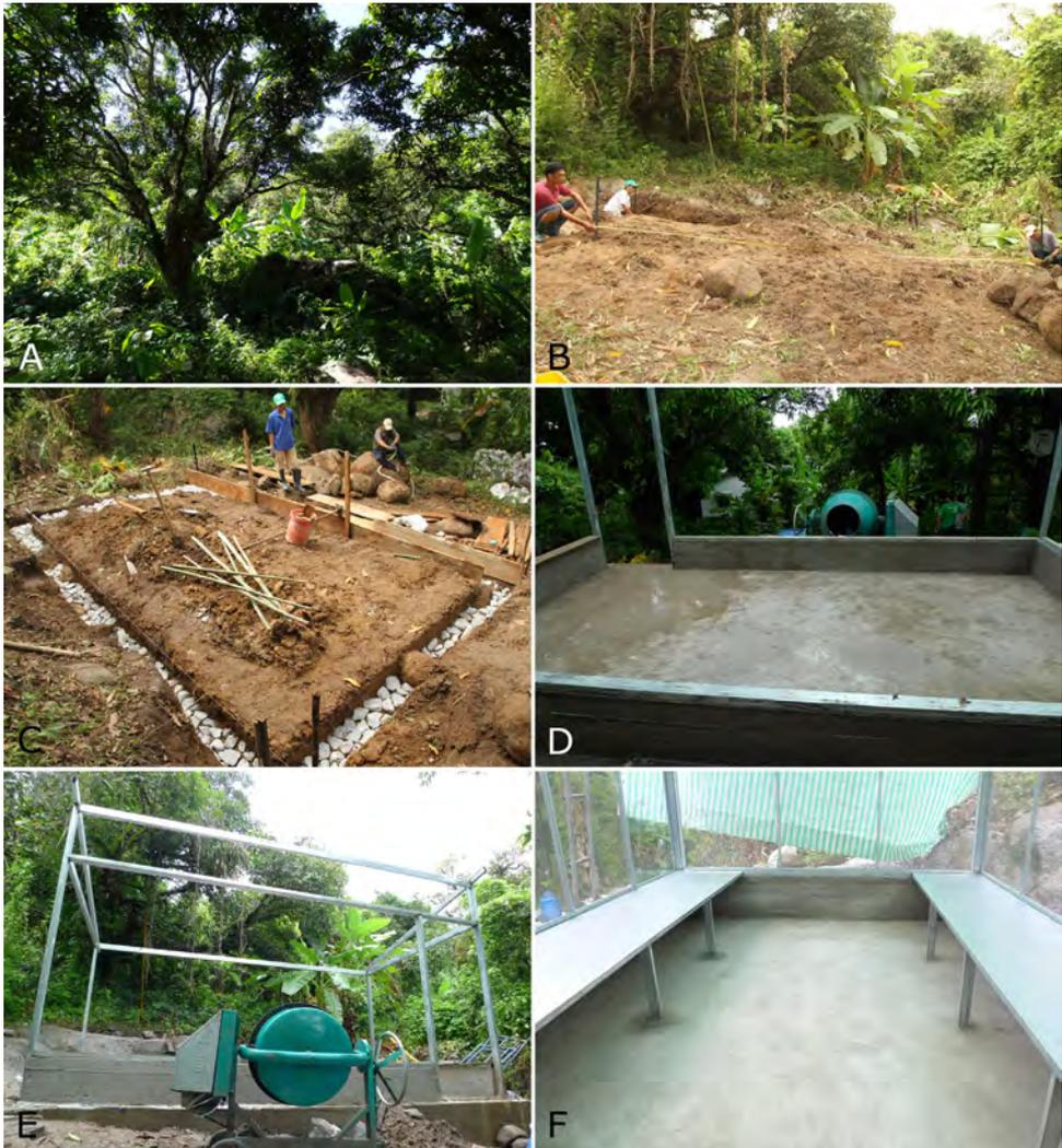
**Fig. 3.** Building phase 1: (A) This part of the Hon Me Station was selected for the building of the gecko house (phot. A. Rauhaus), (B) measuring and marking the cleared site, (C) starting with the fundement, (D) base plate and walls, (E) insertion of iron frames, (F) insertion of tables for the terraria. Photos: K.V. Nguyen.
